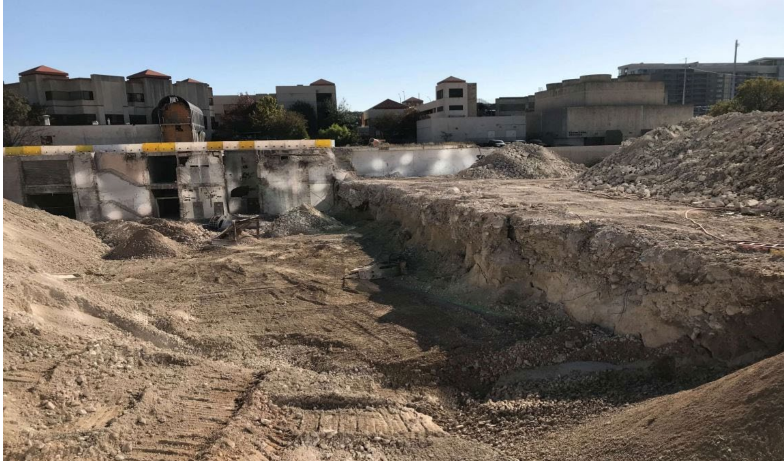
View looking East towards Interstate 35
