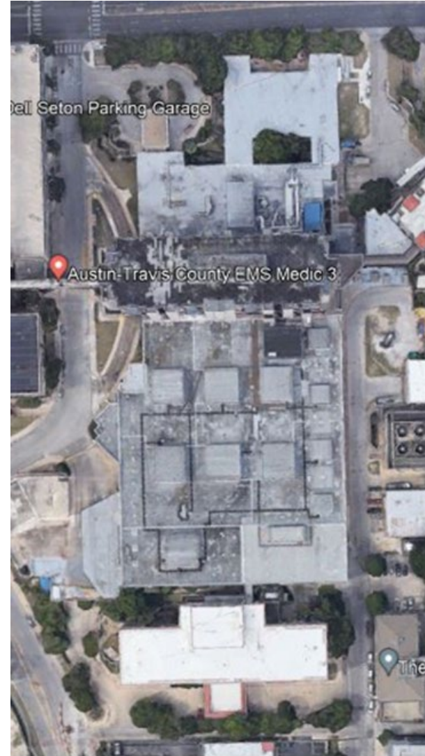
Brackenridge Campus, Pre-Demolition
